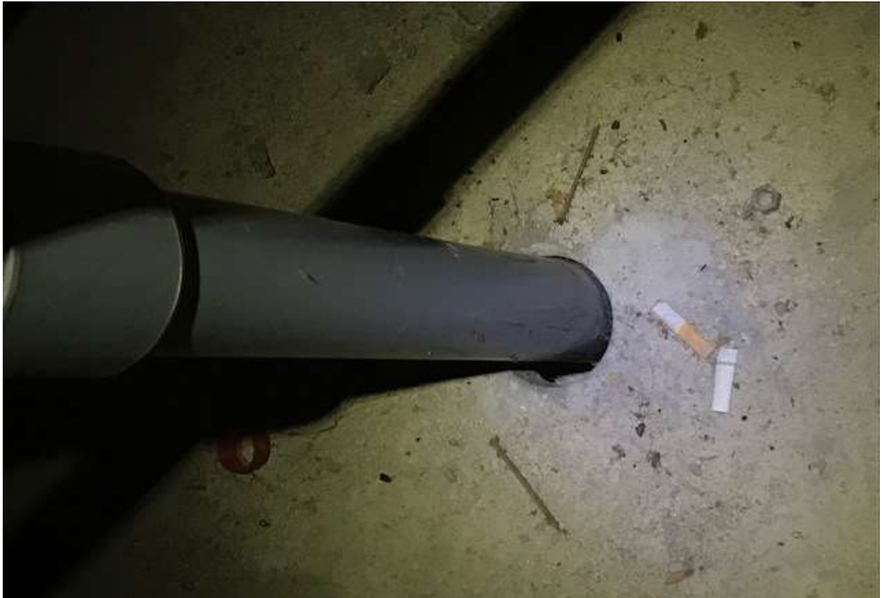
Figure 2 - Pipe Penetration through upper concrete ceiling assembly
