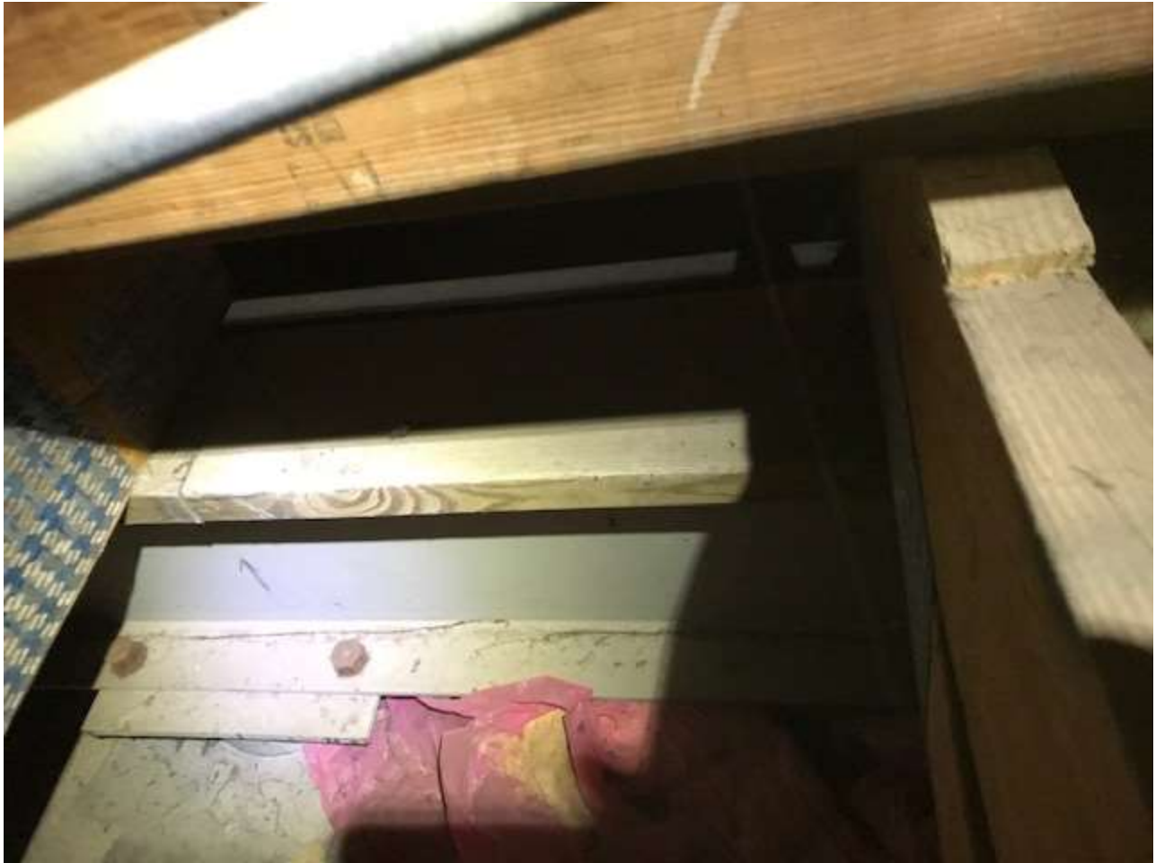
Figure 5 - Steel beam carrying truss reactions - ceiling intact
