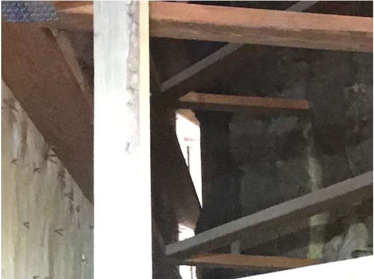
Figure 4 - Heel blocking missing
