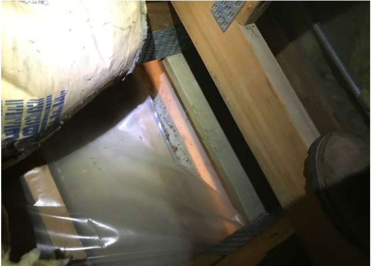
Figure 1 - Ceiling separation from truss structure
