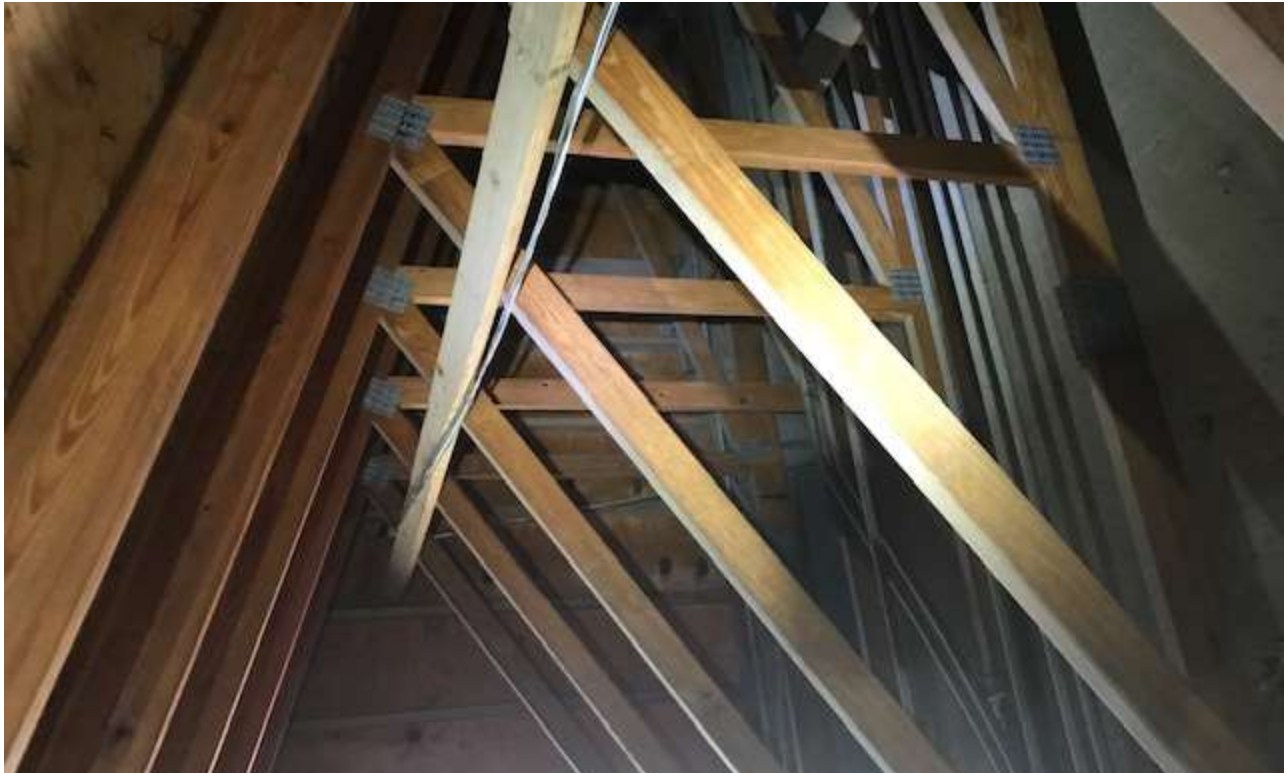
Figure 3 - Gable end bracing and heel blocking missing
