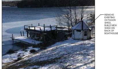
PHOTOS OF BOATHOUSE – REMOVE STAIRS & ROOF DECK. REMOVE OCTAGON SHED
