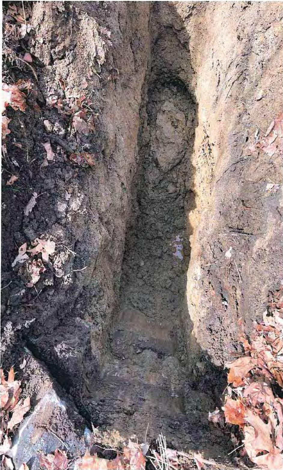
Figure 1: View of test hole #1, groundwater found 4'-0" below the existing top grade.
