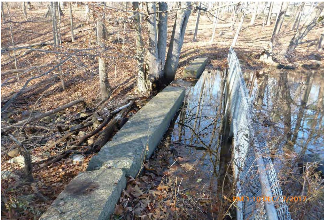
Photo 3 Dam ID# 231-4784 Teakettle Spout Lake Dam 12/07/2017 Concrete non-overflow sections and spillway weir.
