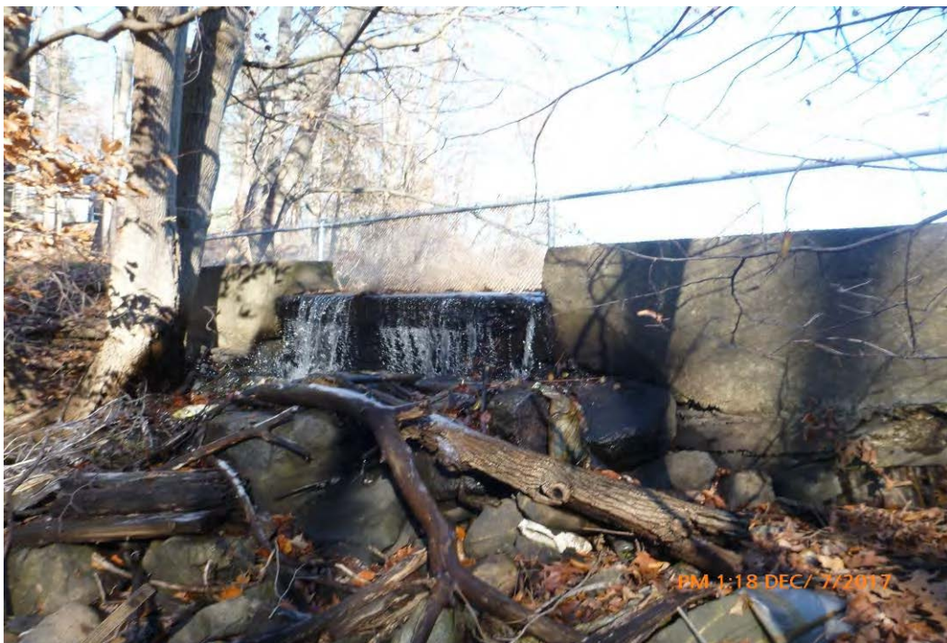
Photo 8 Dam ID# 231-4784 Teakettle Spout Lake Dam 12/07/2017 Downstream view of service spillway and non-overflow sections.
