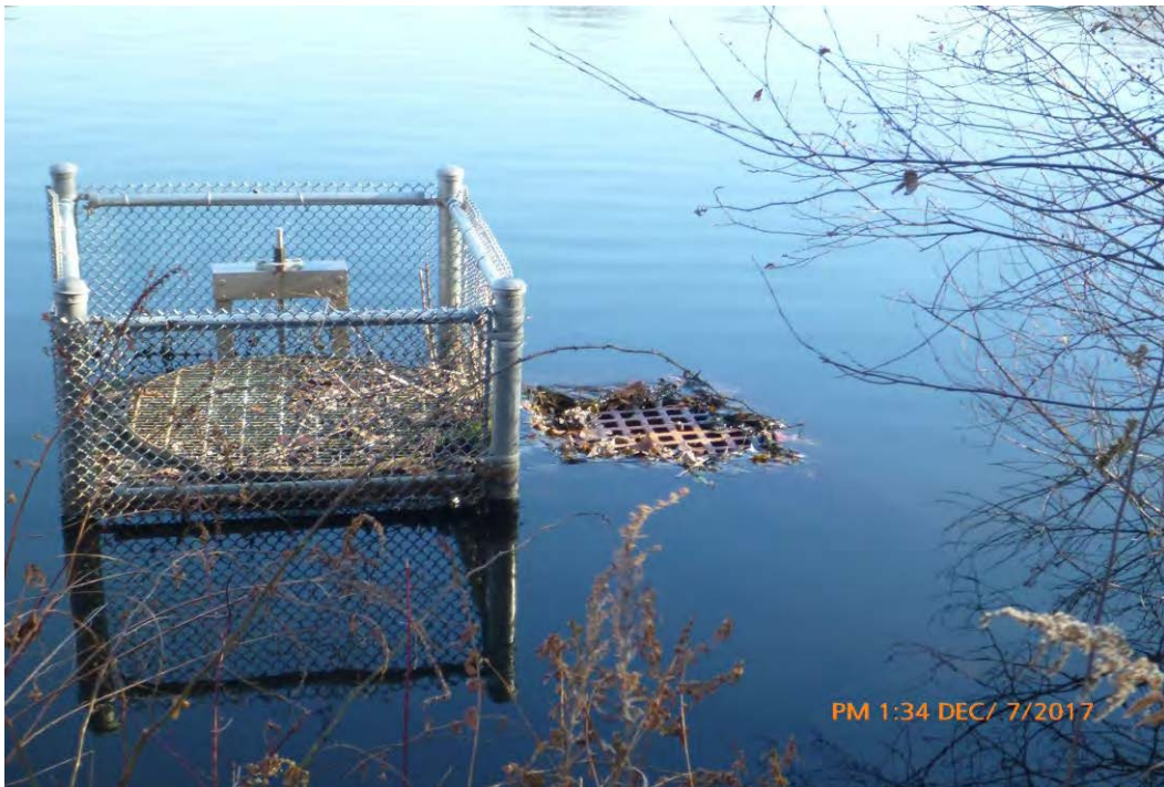
Photo 2 Dam ID# 231-1406 Upper Teakettle Spout Lake Dam 12/07/2017 Service spillway and auxiliary spillway riser inlets.
