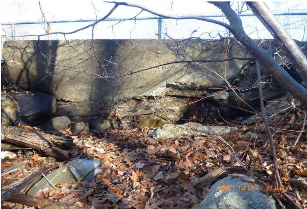
Photo 7 Dam ID# 231-4784 Teakettle Spout Lake Dam 12/07/2017 Concrete deterioration and voids on downstream left non-overflow section.
