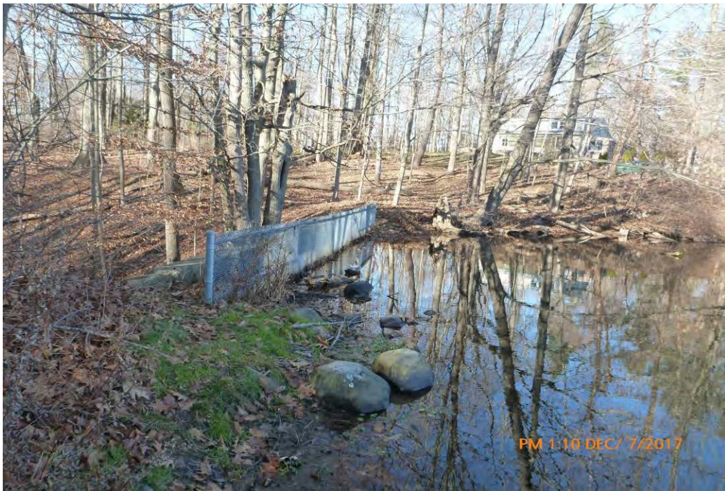
Photo 2 Dam ID# 231-4784 Teakettle Spout Lake Dam 12/07/2017 Fish screen upstream of service spillway.
