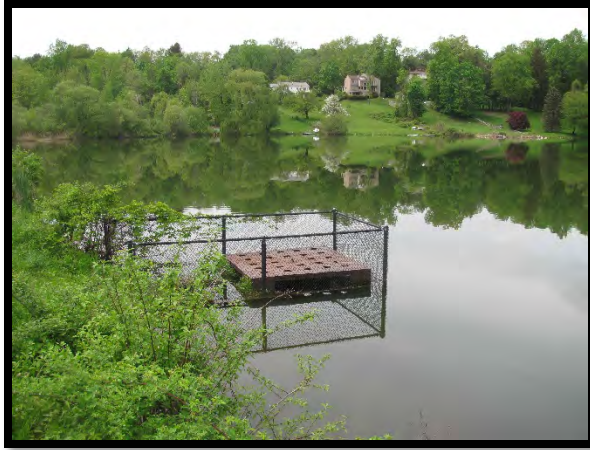
Metal grate orifice opening on east side of riser
