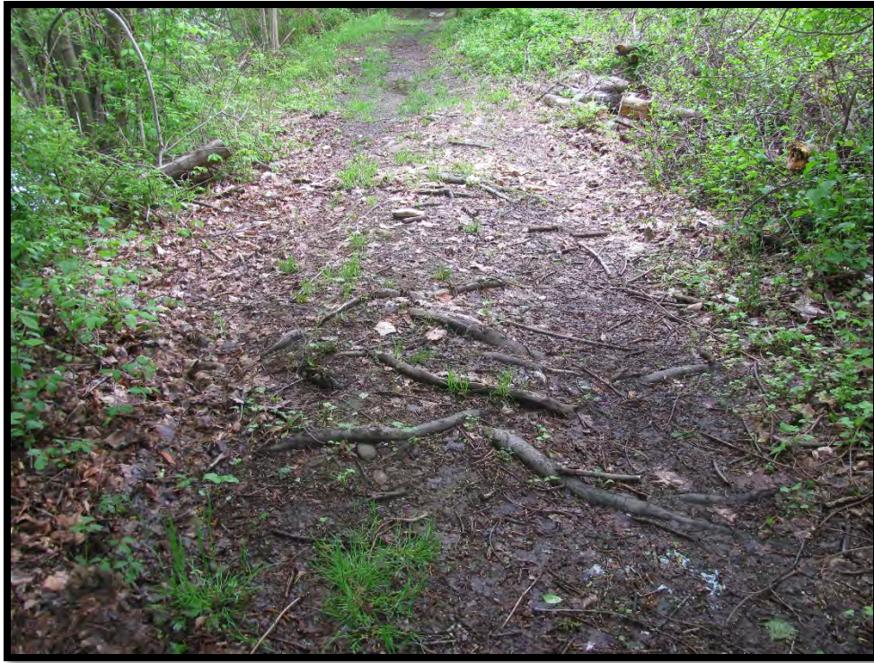
Photo P-9 Trees roots along dam crest; view north
