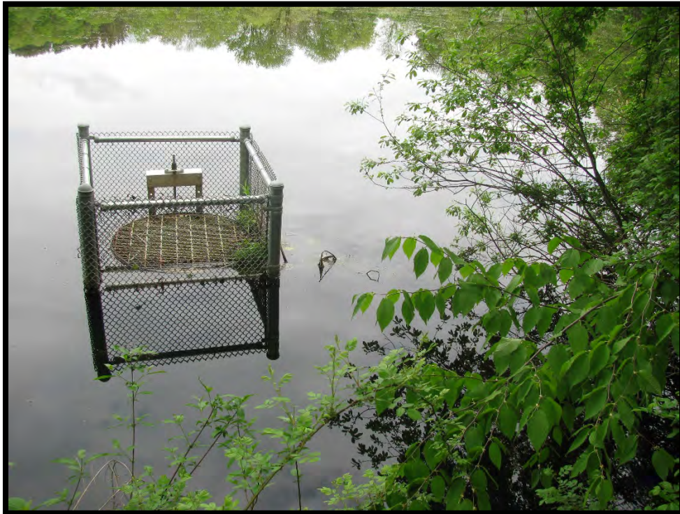
Photo P-8 Auxiliary Riser inlet grate and fencing; view east
