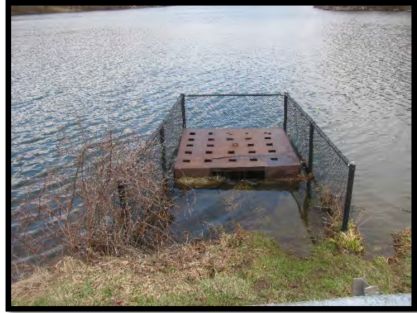
Metal grate orifice opening on north side of riser
