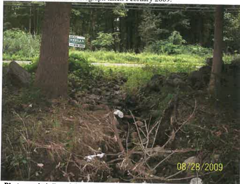
Photograph 4: Breech in stone wall with erosional swale starting at ditch along Drewville Road. View is to the south/southeast. Photograph taken August 2009.
