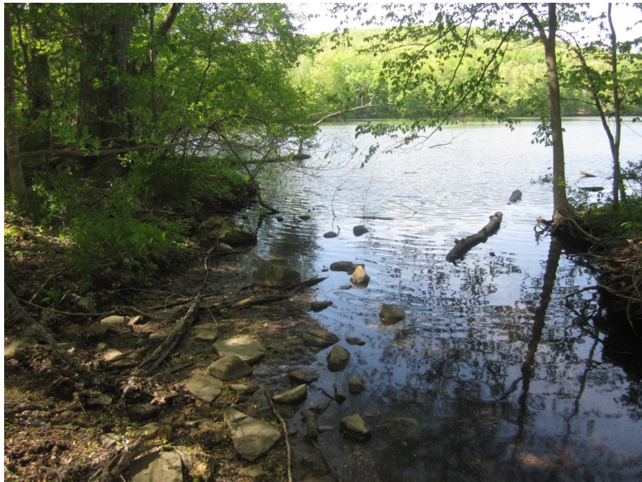
Photograph 8: Reservoir erosion. Photograph taken June, 2015.
