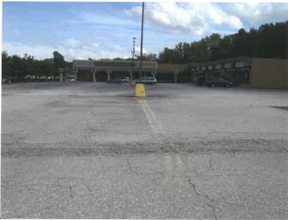
Photograph 1. Representative view of existing commercial building facing southeast.
