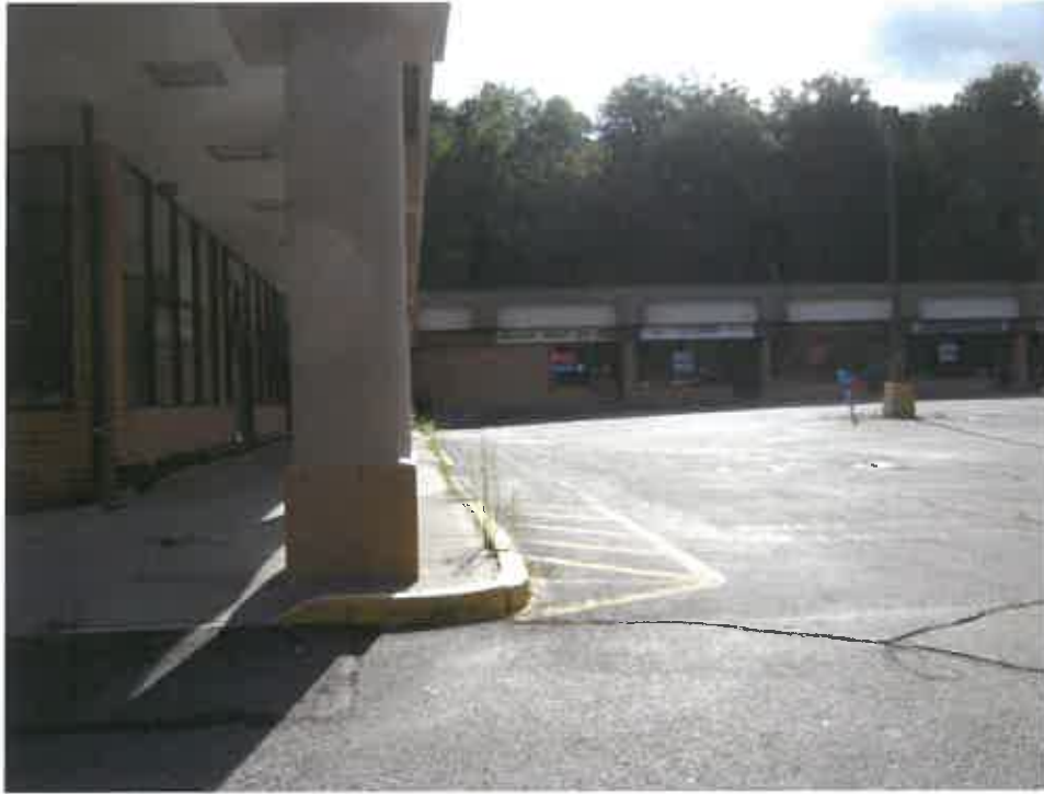
Photograph 7. Representative view of north side of commercial building facing southwest.
