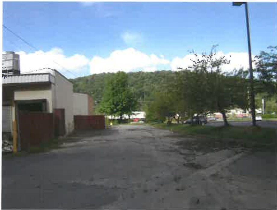
Photograph 4. Representative view of south side of commercial building facing northeast.
