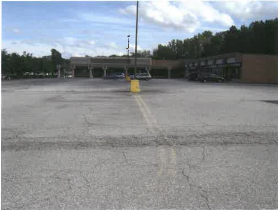
Photograph 1. Representative view of existing commercial building facing southeast.
