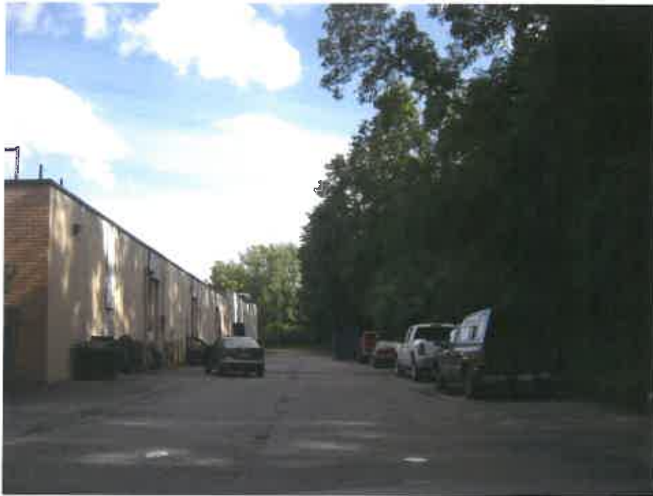
Photograph 2. Representative rear view of existing commercial building facing southeast.
