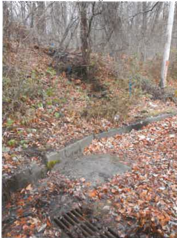
Photograph 10: Representative view of the intermittent watercourse (marked by blue ribbons) dispersing into catch basin, facing northwest.
