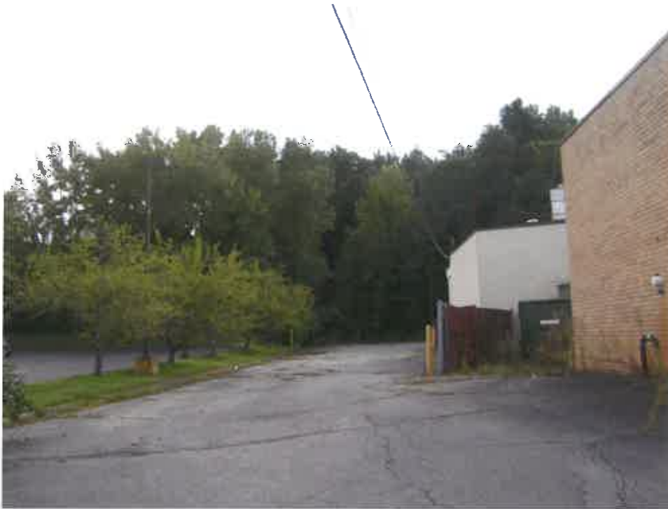
Photograph 5. Representative view of south side of commercial building facing southwest.
