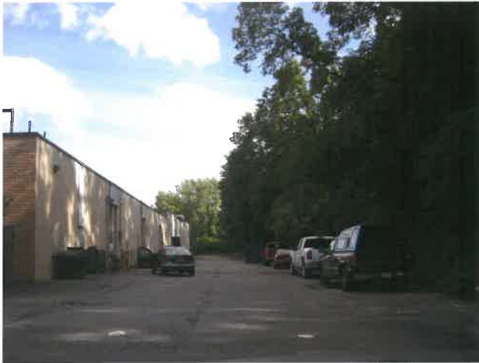
Photograph 2. Representative rear view of existing commercial building facing southeast.
