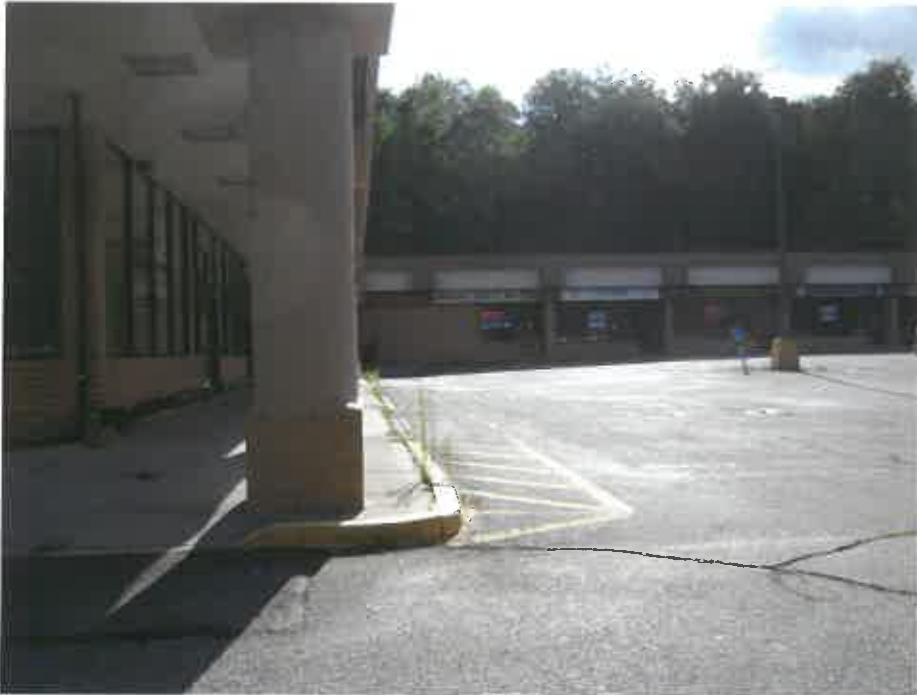
Photograph 7. Representative view of north side of commercial building facing southwest.
