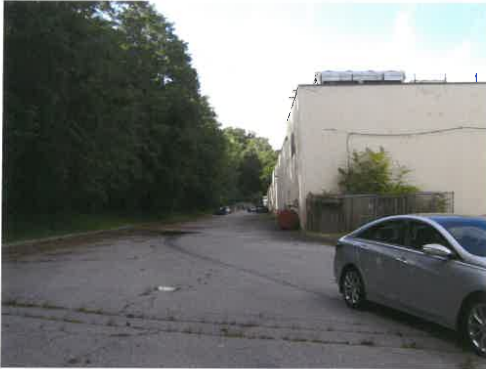
Photograph 3. Representative view of rear of commercial building facing northwest.
