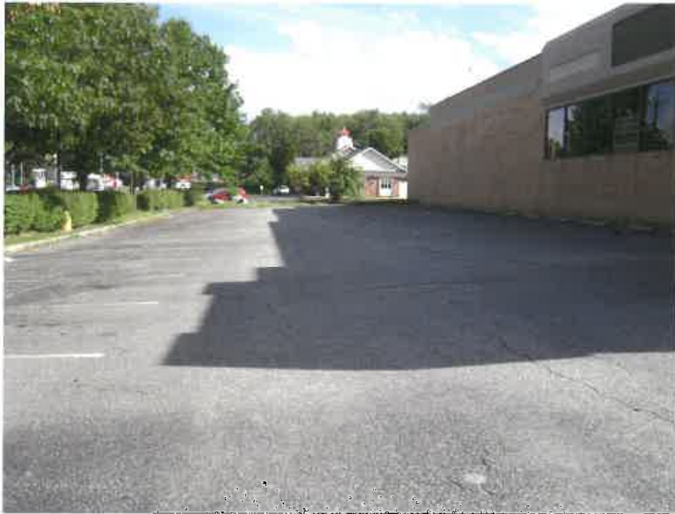
Photograph 6. Representative view of northeast side of commercial building facing southeast.
