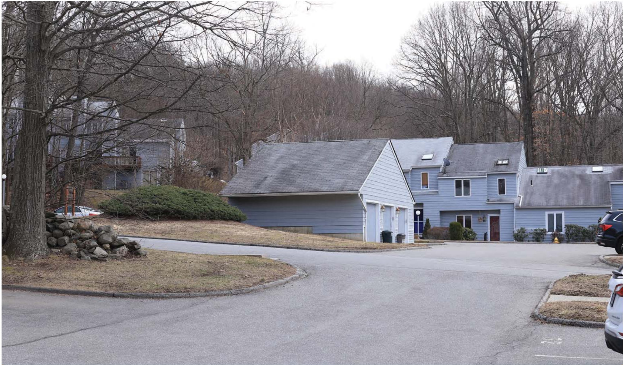
Existing Condition VP7 - Maple Drive near #66
