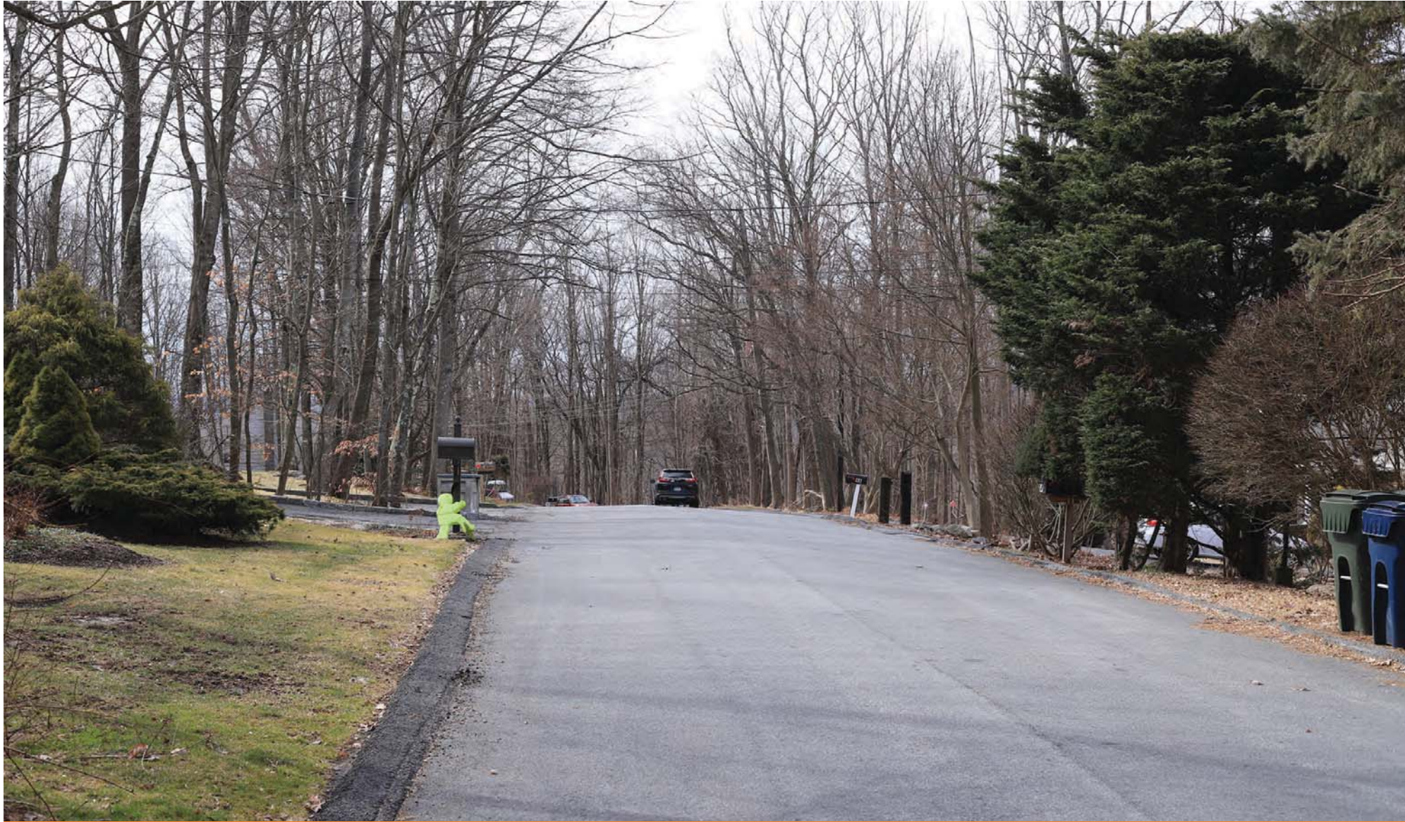
Existing Condition VP12 - Walton Drive near #43
