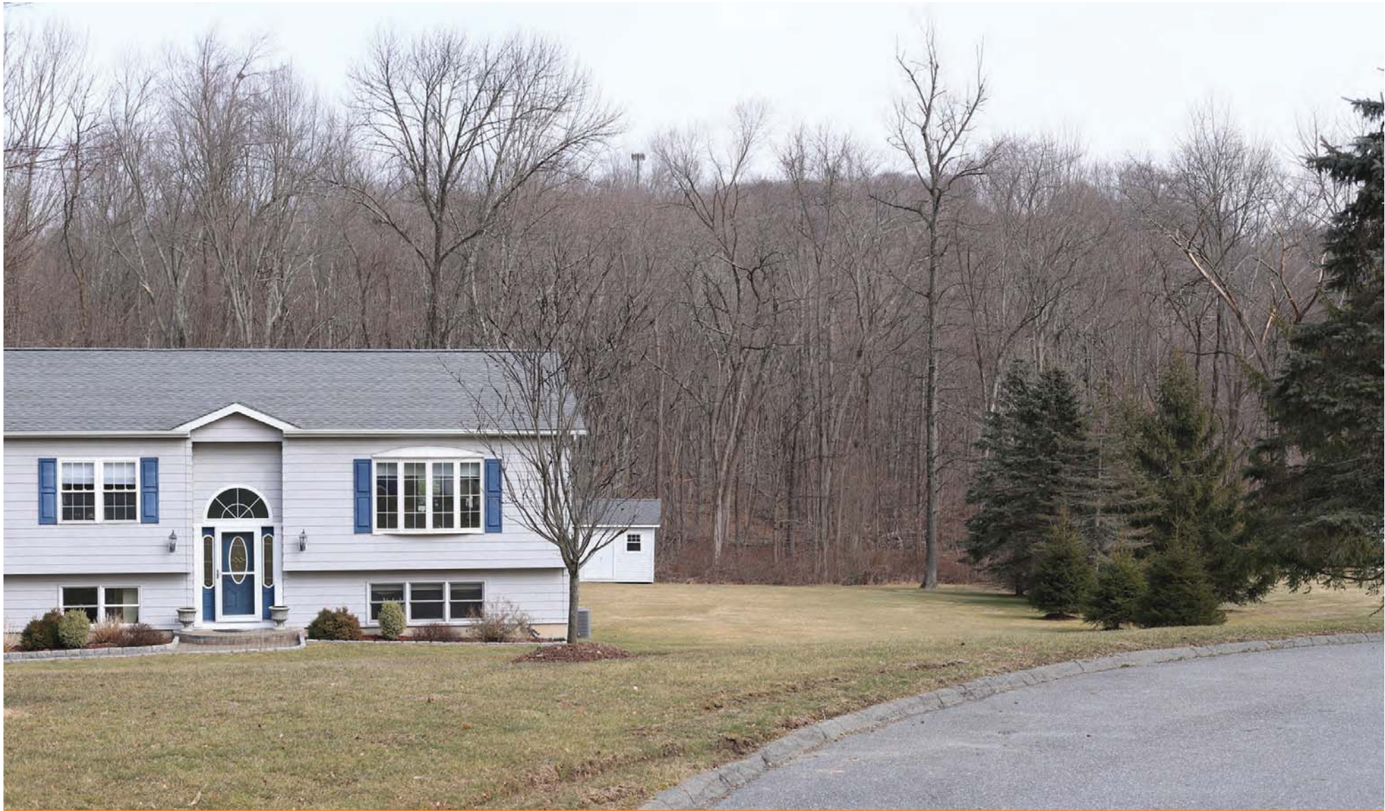
Simulated Condition - 140 ft Monopole Tower - Brown Color Alternative VP3 - Fassitt Drive near #61
