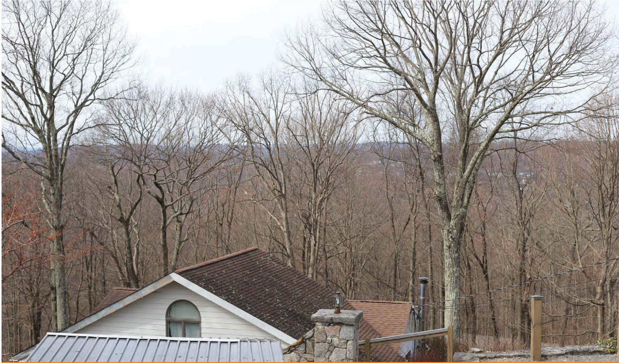
Existing Condition VP14 - Summit Circle Drive at cul-de-sac
