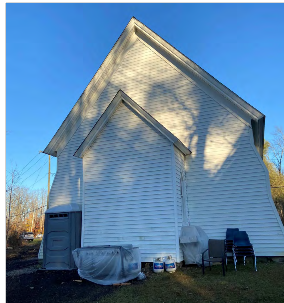
REAR VIEW OF CHURCH (WEST)
