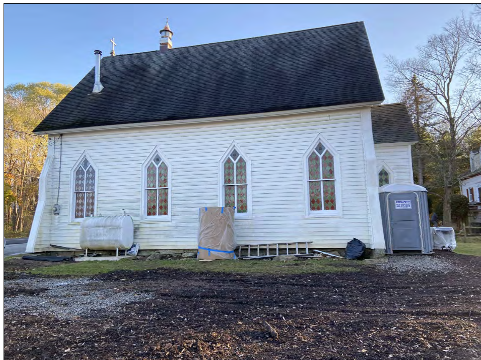
RIGHT VIEW OF CHURCH (NORTH)
