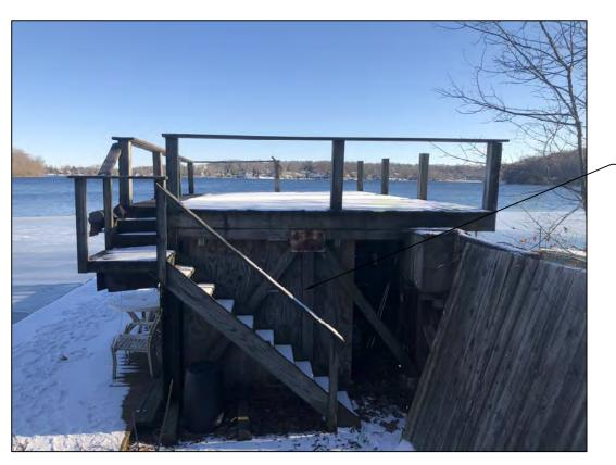
REMOVE EXISTING STAIRS AND ROOF RAILING. INSTALL **NEW PEAKED** ROOF. INSTALL NEW 4'-0" X 11'-9" SHED AT BACK OF BOATHOUSE ON EXISTING CONCRETE PLATFORM.
