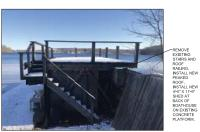
PHOTOS OF BOATHOUSE - REMOVE STAIRS & ROOF DECK. REMOVE OCTAGON SHED
