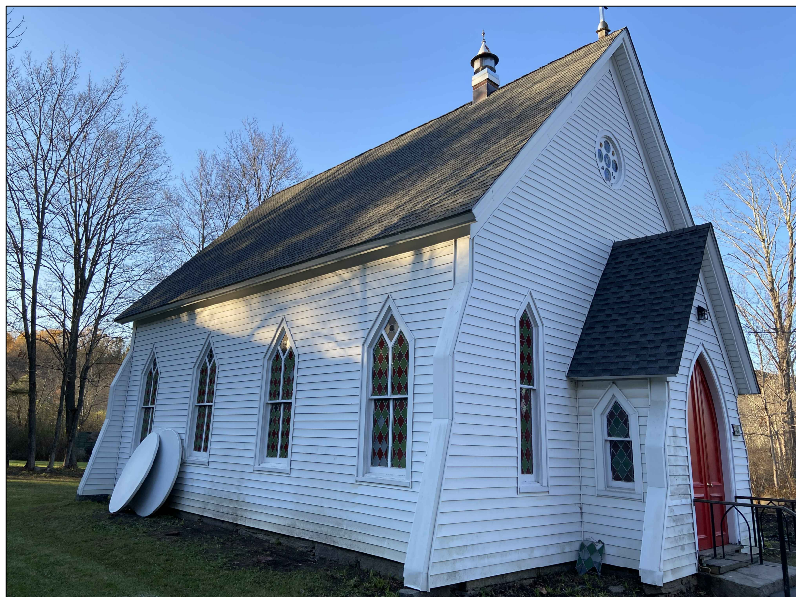
FRONT LEFT VIEW OF CHURCH (SOUTH)
