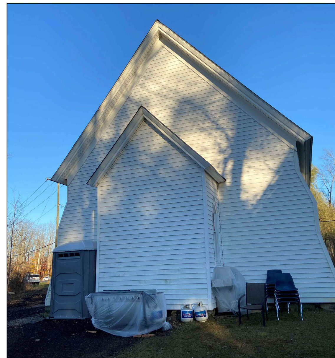
REAR VIEW OF CHURCH (WEST)
