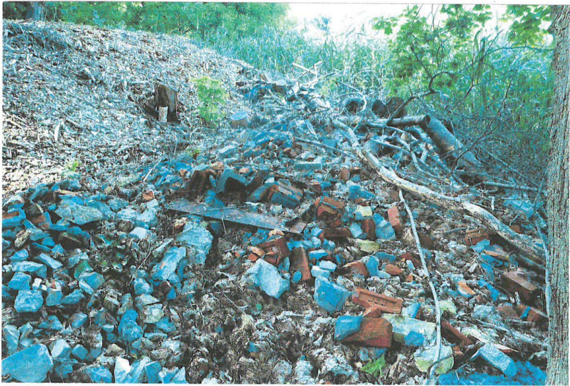
Photo 6 Looking north and across slope of fill material on the eastern edge of the site. Note dumped brick, concrete, and asphalt fragments; dumped and spread woodchips in upper left corner of the photo.
