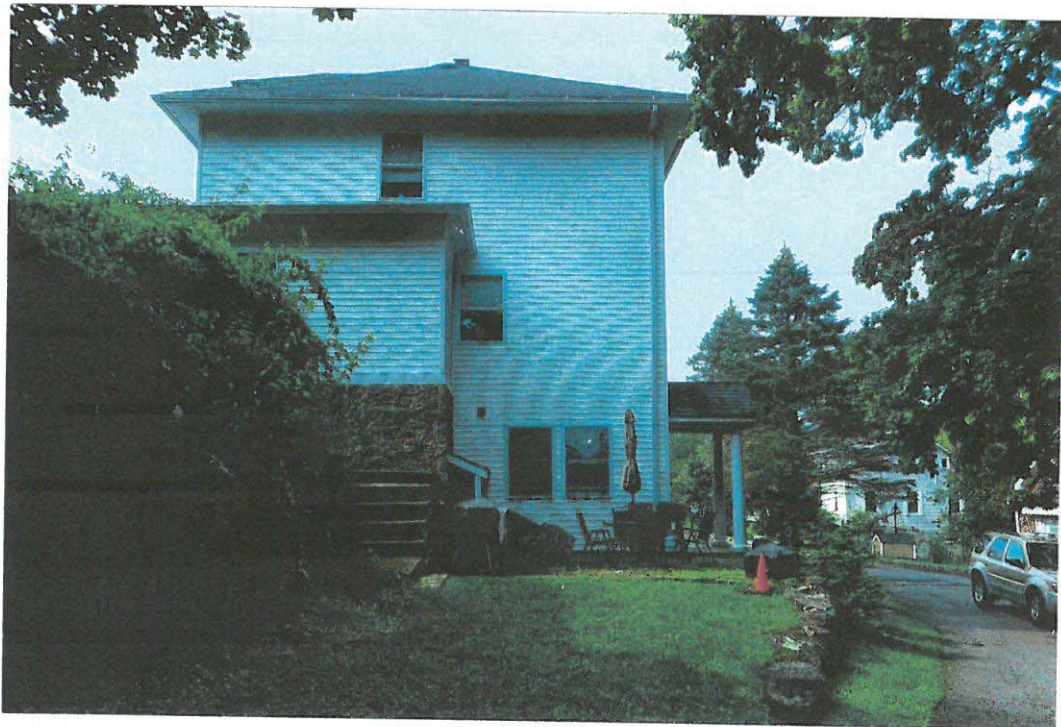
Photo 2 Looking north toward south side of building.
