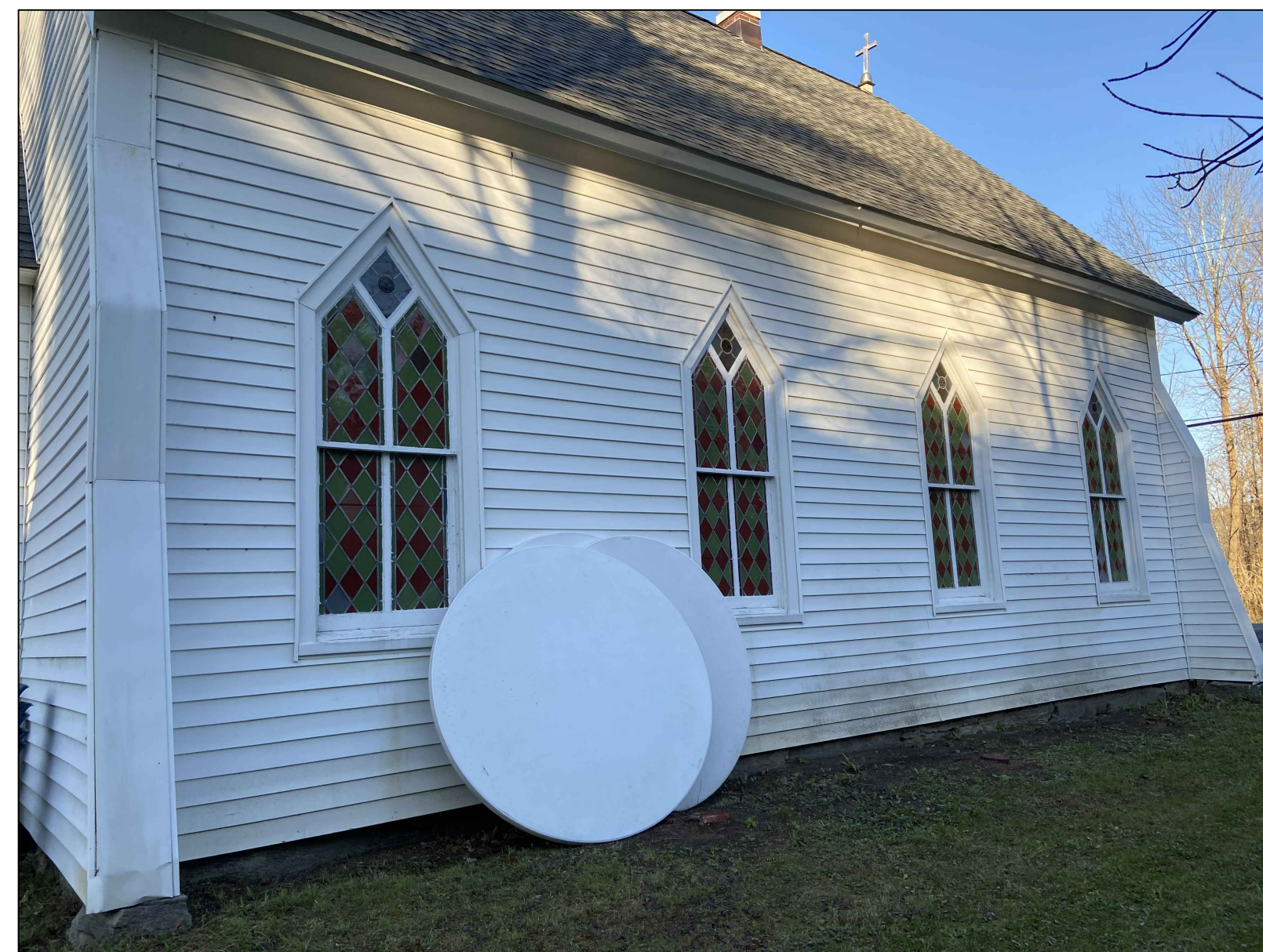
LEFT VIEW OF CHURCH (SOUTH)
