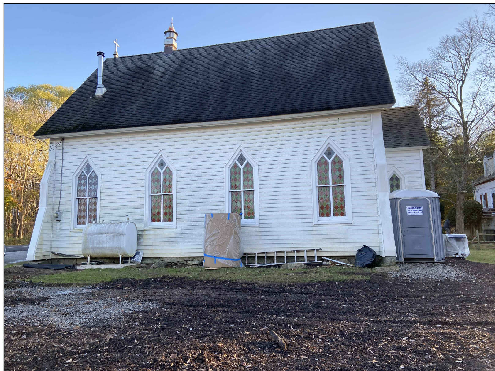
RIGHT VIEW OF CHURCH (NORTH)
