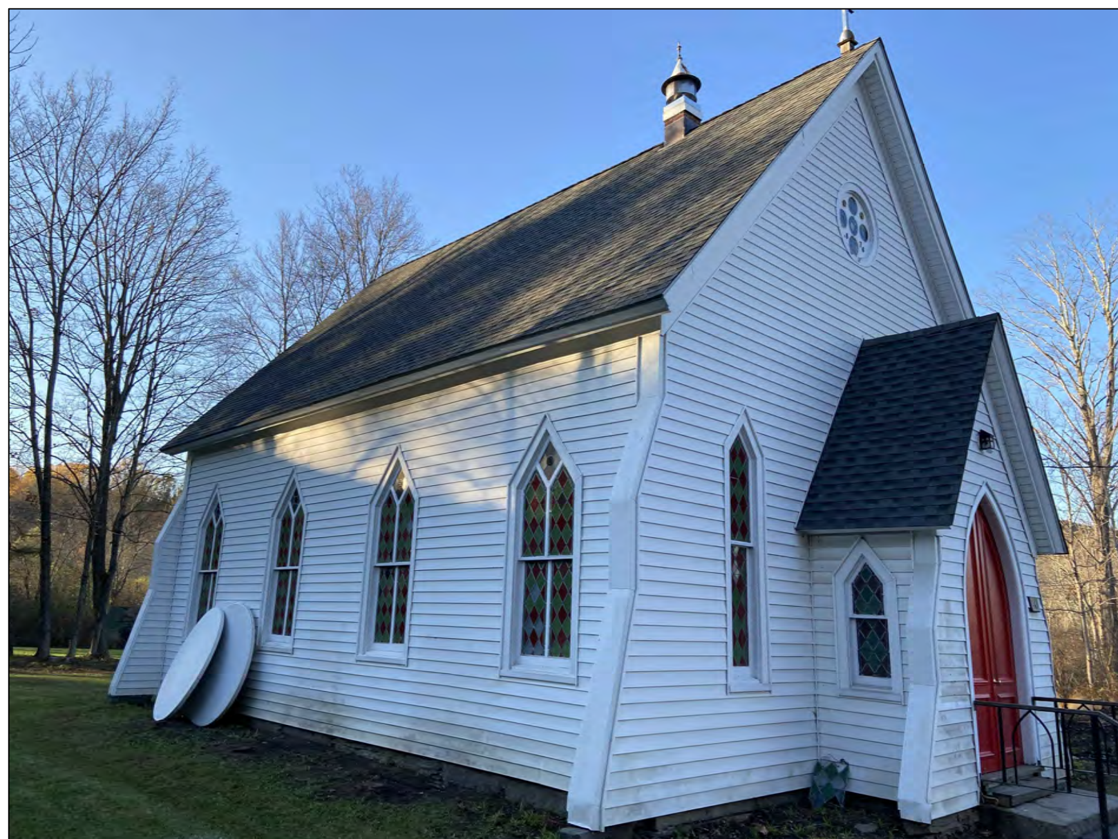
FRONT LEFT VIEW OF CHURCH (SOUTH)
