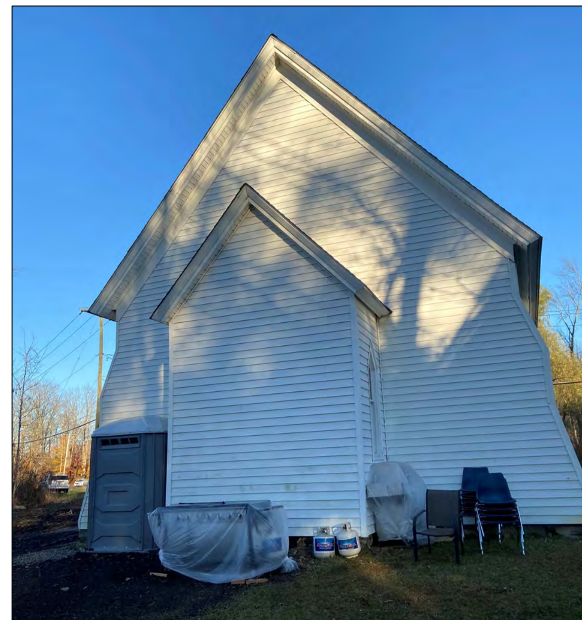
REAR VIEW OF CHURCH (WEST)
