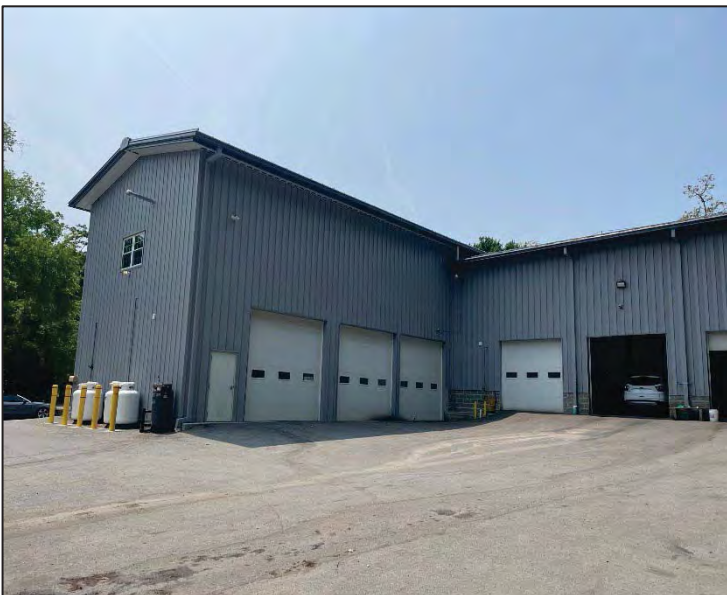
Photo 23 – View of the auto repair shop located adjacent to the southwestern portion of the Subject Property
