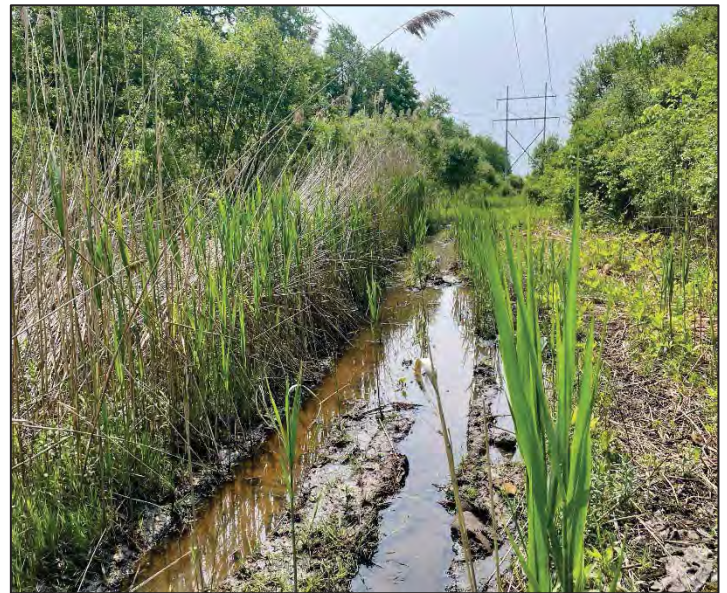
Photo 4 – View of standing water along the utility easement located on the northeastern portion of the Subject Property
