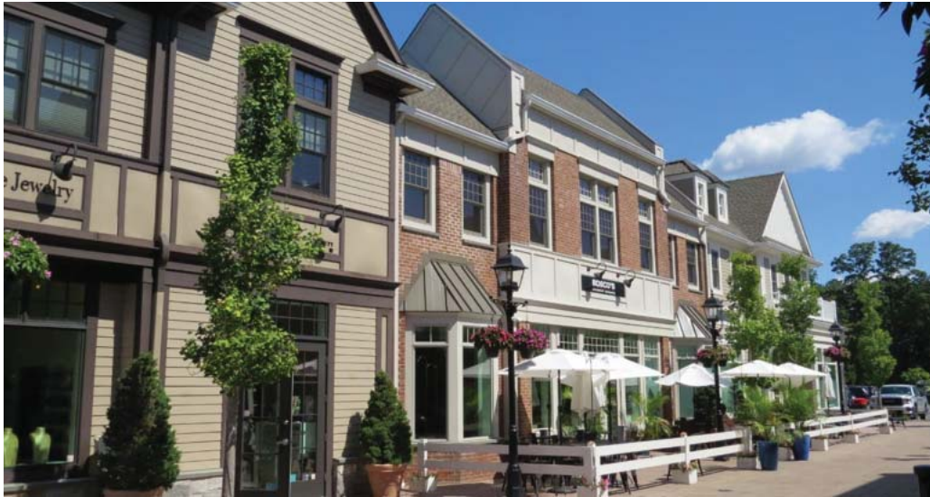
An infill project in Armonk, NY. Although one building, the massing is broken in size and massing to give the appearance of multiple buildings. Building heights are two stories, and large shop windows provide visual interest.
