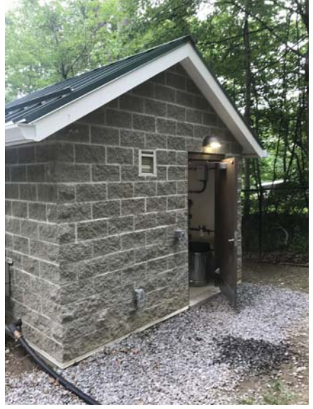
③ Close Up of Existing Building SCALE: NO SCALE
