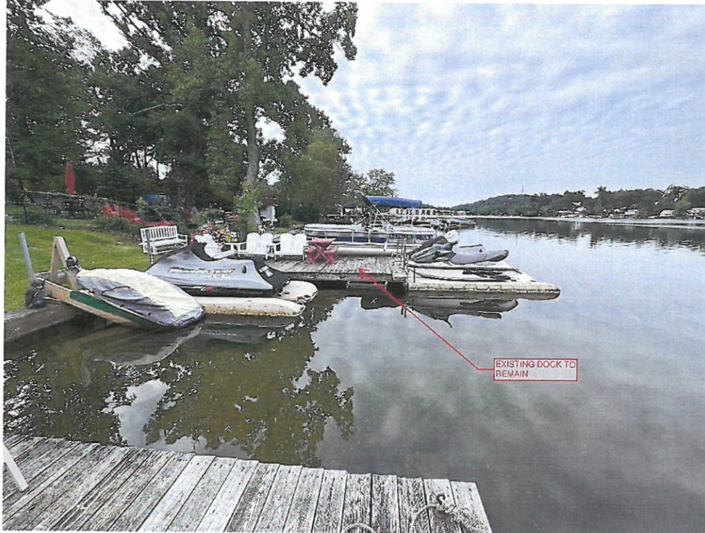
Figure 7: Existing Dock to Remain.
