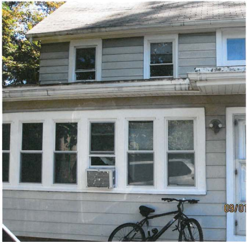
Building Front View
