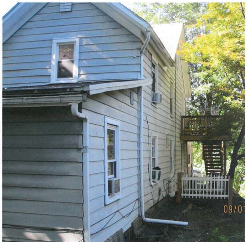
Building Left Side View
