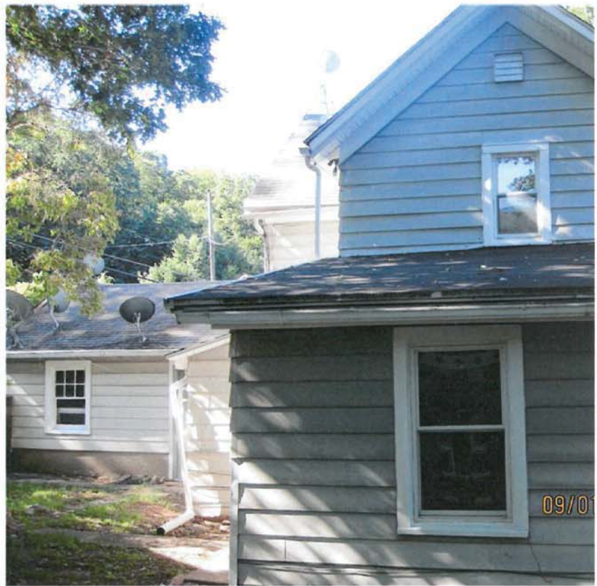
Building Back View
