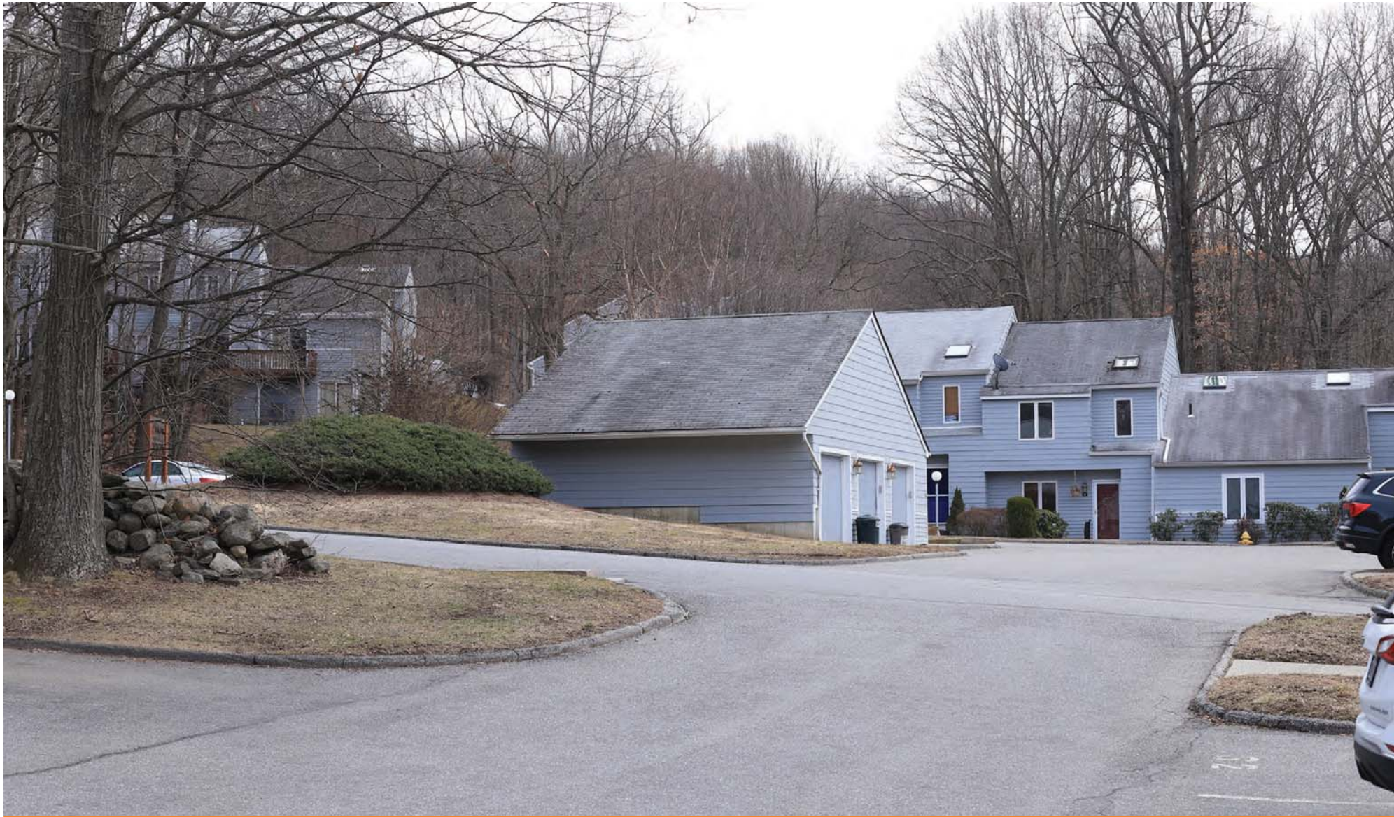
Existing Condition VP7 - Maple Drive near #66
