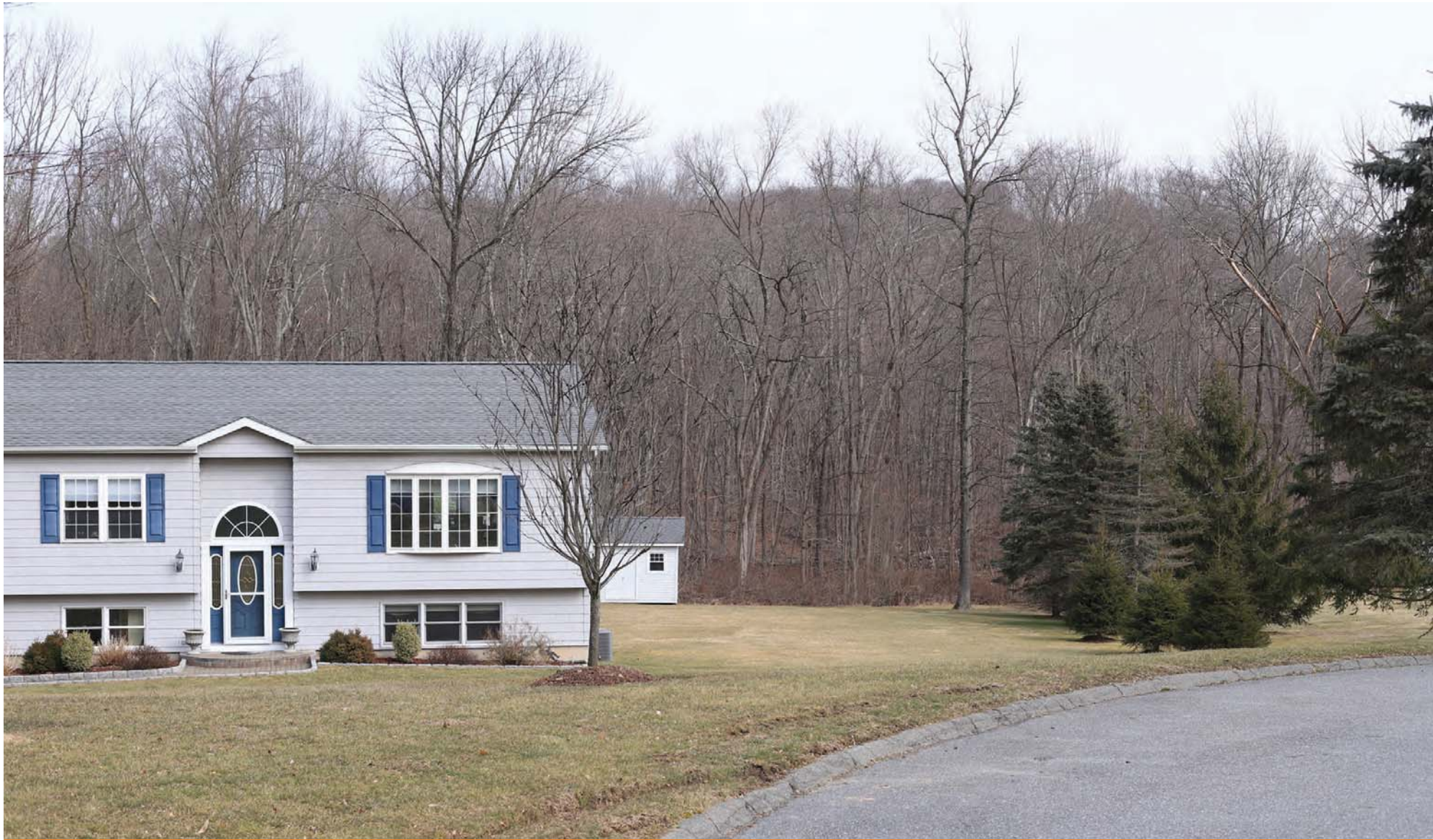
Existing Condition VP3 - Fassitt Drive near #61
