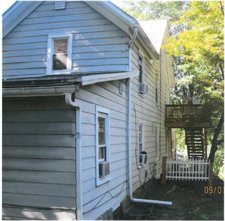
Building Left Side View
