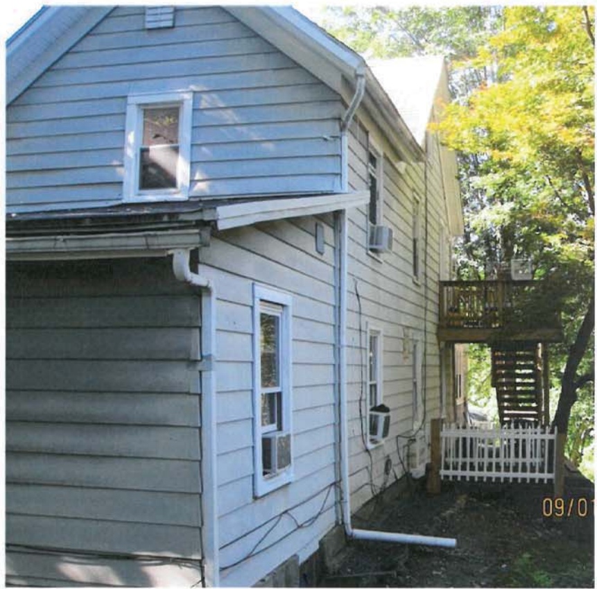
Building Left Side View
