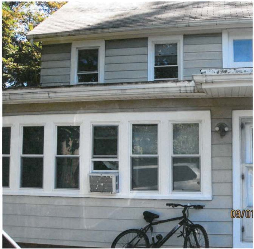
Building Front View
