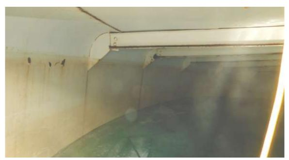
Top photo shows the interior roof lap seams, which appear to be in good condition.
