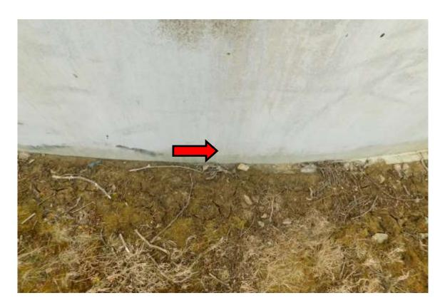
Photo shows the tank has no grounding system. We recommend electrically grounding the tank for lightning protection as required by OSH Act of 1970 Section 5.
