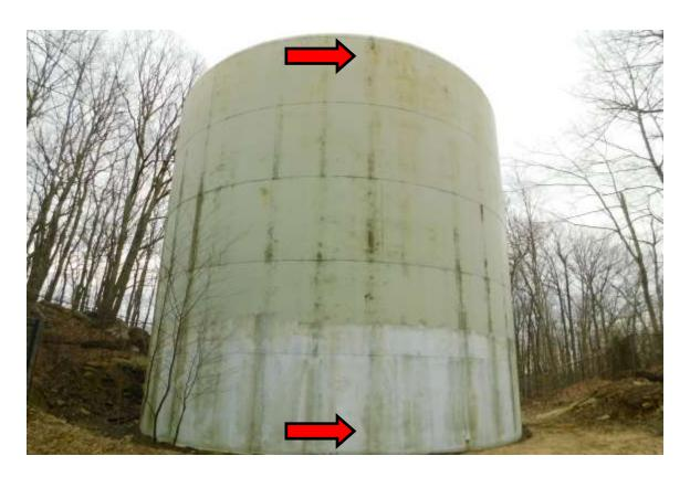
Photo shows the tank is not equipped with a liquid level indicator. We recommend installing a float-type liquid level indicator.
