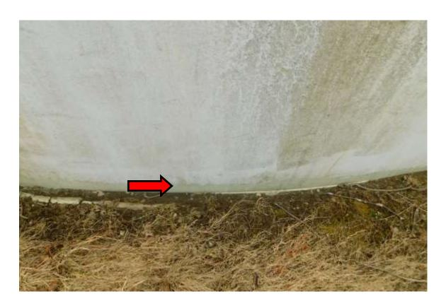
Photo shows the condition of the shell. Currently there is no drain valve. We recommend installing a frost proof drain valve near the shell-to-floor connection, complete with a locking device to prevent unauthorized draining of the tank and a splash pad to direct water away from the foundation.
