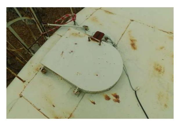
Photo shows the condition of the 25" x 35" primary roof hatch. Roof openings on this tank require the following to be in compliance with AWWA D100-11; 7.4.3 Roof openings and OSHA 1910.146(c)(2) Confined spaces.
