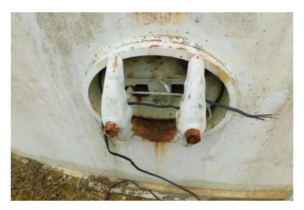
Photo shows the condition of the 18" x 24" primary shell manway. The following is required for the tank to be in compliance with AWWA D100-11; 7.4.4 Shell manholes and OSHA 1910.146(c)(2) Confined spaces.
