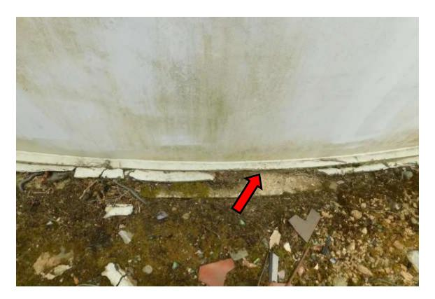
Photo shows the condition of the foundation. We recommend repairing any cracks and spalling in the concrete with a commercial non-shrinking grout, caulking/grouting around the base of the tank to foundation connection to prevent water from entering under the tank, then sealing the foundation with a sealant.
