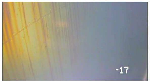
Photos show the condition of the interior coating system. We recommend sand-blasting all rusted and abraded interior areas to SSPC-SP10 (near white), and brush blasting all remaining interior areas to SSPC-SP7; then applying one (1) spot coat of epoxy primer to all areas sandblasted to #10, stripe coating all weld seams, and applying epoxy to the entire tank, to achieve 8 to 10 mils of total dry film thickness. Total mil thickness will include a combination of the existing and new coating.
