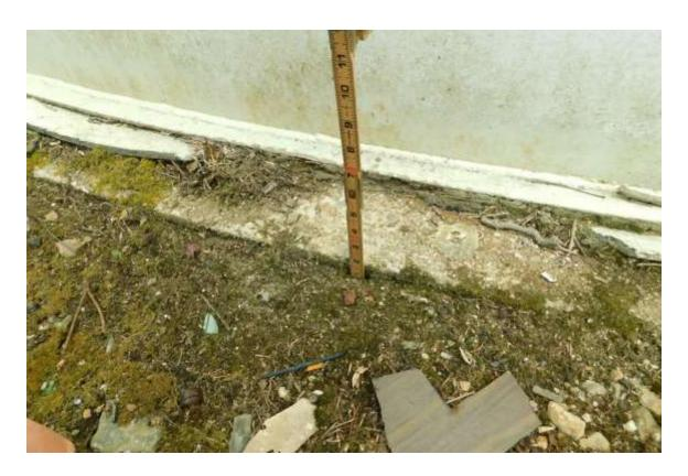
Photo shows the condition of the foundation. AWWA D100-11; 12.7.1 Height aboveground states, "The tops of the concrete foundations shall be a minimum of 6" above the finished grade, unless otherwise specified." We recommend clearing any dirt, debris and other loose gravel away from the tank foundation, down to a minimum 6" below top of foundation. This should be done by a local excavating company.
