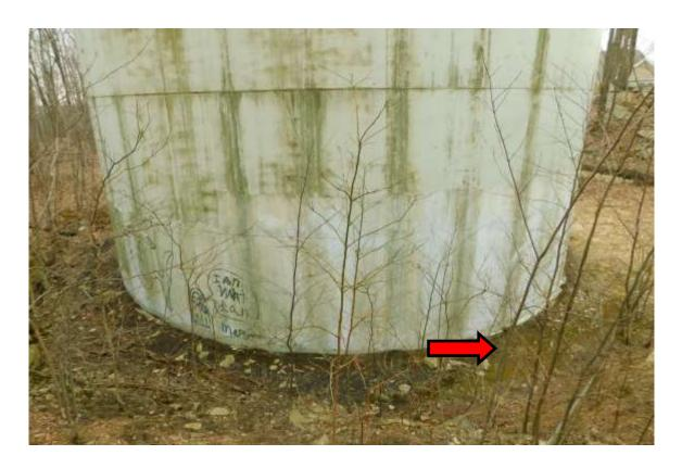
Photo shows the condition of the tank site. **Notice the vegetation growth around the tank foundation.** This could lead to deterioration of the structural components of the tank. OSHA 1910.176(c) states, "Storage areas shall be kept free from accumulation of materials that constitute hazards from tripping, fire, explosion, or pest harborage. Vegetation control will be exercised when necessary." We recommend removing the vegetation from around the tank foundation. This should be done by others.
