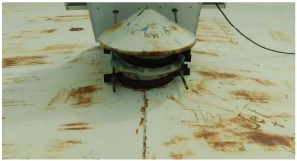
Photos show the condition of the existing 14" roof vent. This vent is allowing the ingress of rain and wind-borne contaminants into the water system. An improperly vented tank may cause external pressure to act on the tank which can cause buckling even at low pressure differential. We recommend replacing the existing roof vent with a vacuum-pressure, frost proof vent and screen.
