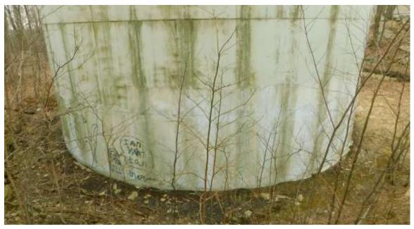
Photos show the tank exterior coating system. We recommend pressure washing the tank exterior with biodegradable detergent injection (minimum 3,500 psi at 3.0 gpm) then removing all loose rust and scale with wire brushes and hand scrapers in accordance with SSPC#2 (hand tool cleaning), spot priming and applying one (1) finish coat of acrylic paint.
